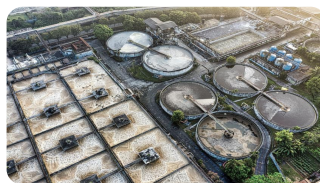
ZLD / MLD Wastewater Treatment
